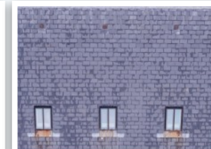
Difficult to access roof surveys even in congested areas
